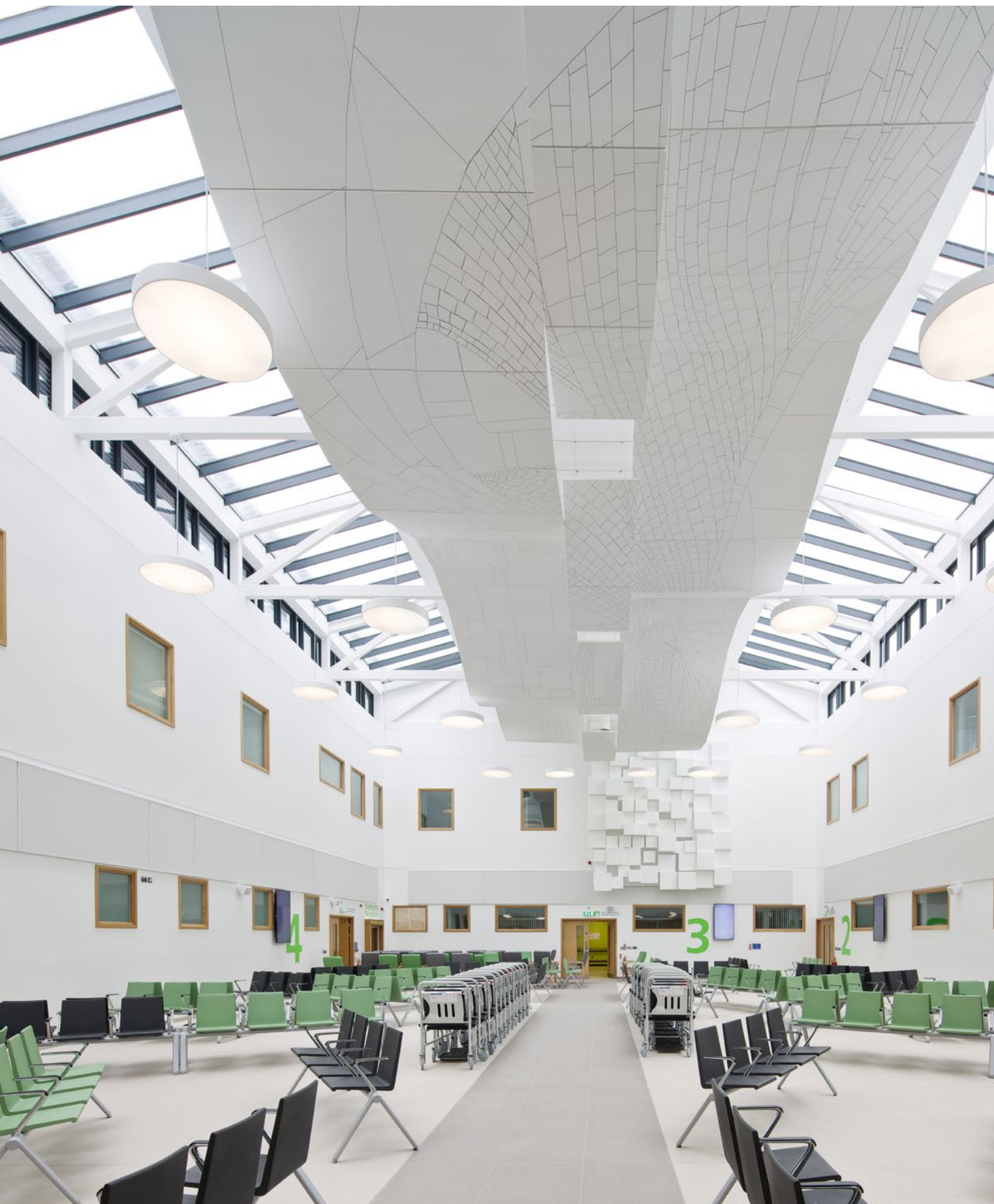
Project Morriston Hospital Product Rockfon Eclipse Customised
