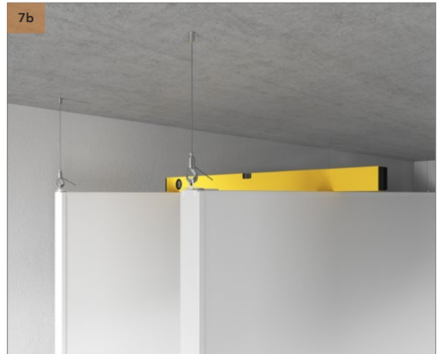
Place a level on top or underneath the baffles to ensure their evenness. Levelling can be done by releasing the lock on the hook and pulling on the wire cable.
