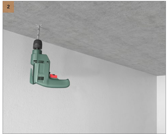
Drill where you have marked drilling points.
